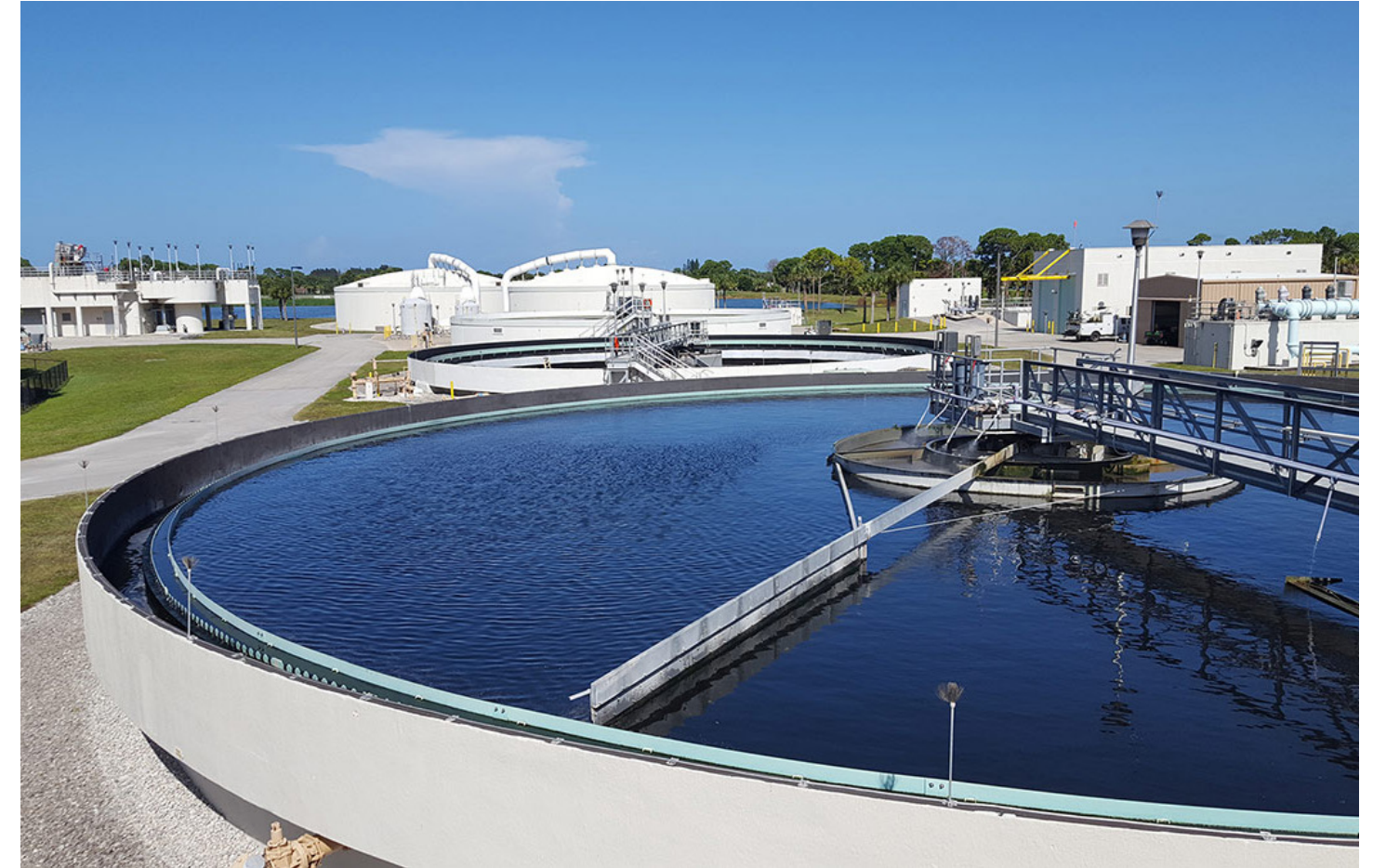
Loxahatchee River Environmental Control District, “Secondary clarifiers,” 2018.
