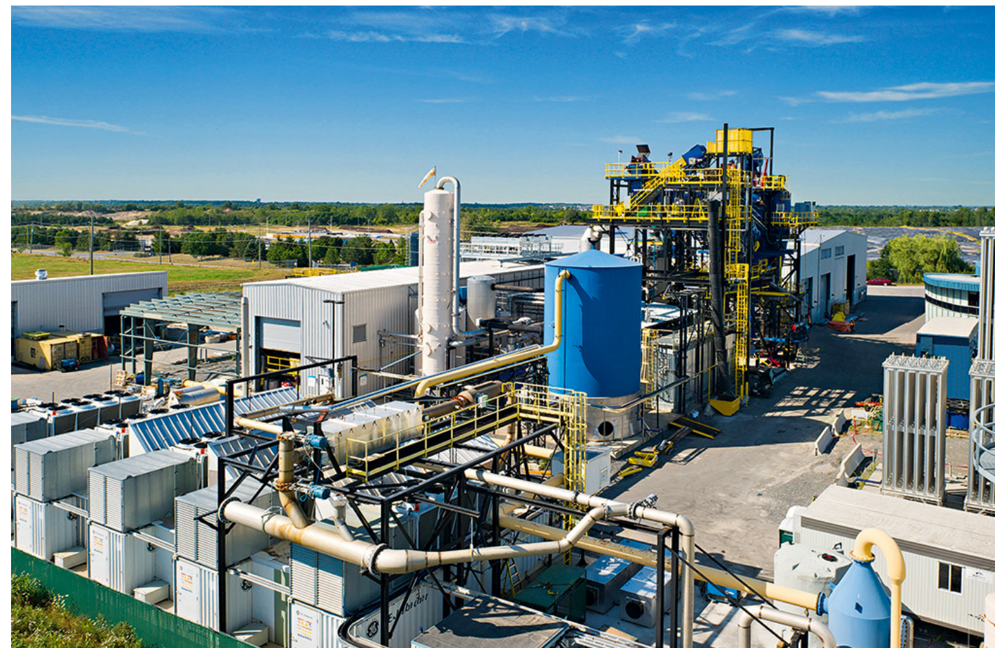
Waste conversion demonstration facility, Plasco Energy Group , 2014.
