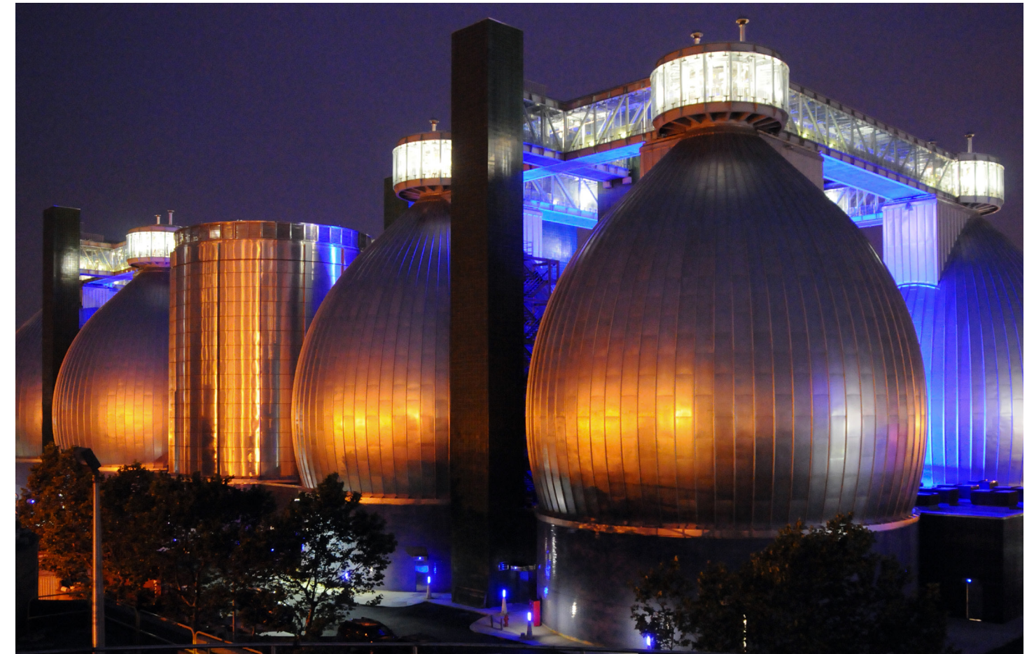
New York Department of Environmental Protection, "Biodigesters," 2014.
