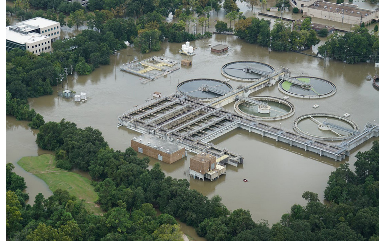
Karl Spencer, "Wastewater treatment plant flooding in Hurricane Harvey," 2018.
