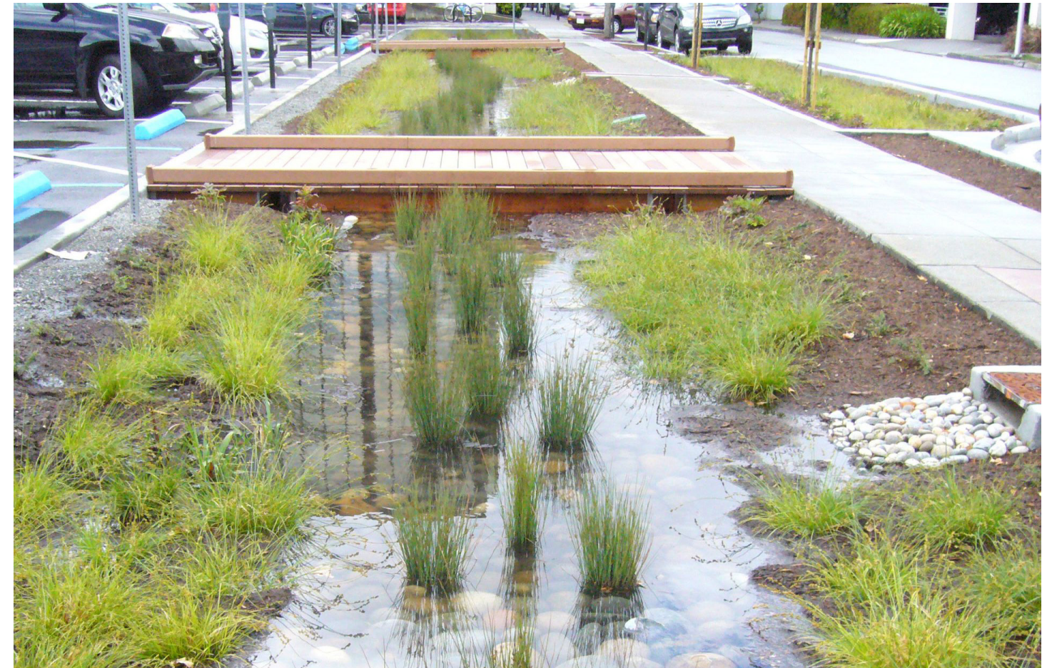
Chesapeake Stormwater Network, "Bioretention in street median in Arlington County", Chesapeake Stormwater Network , 2015
