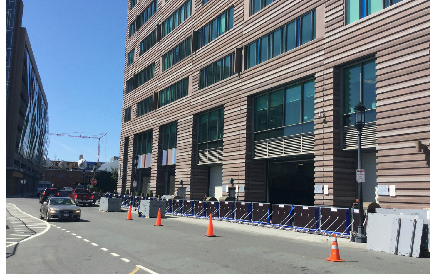
"AquaFence deployed in downtown Boston", Level Infrastructure , 2017
