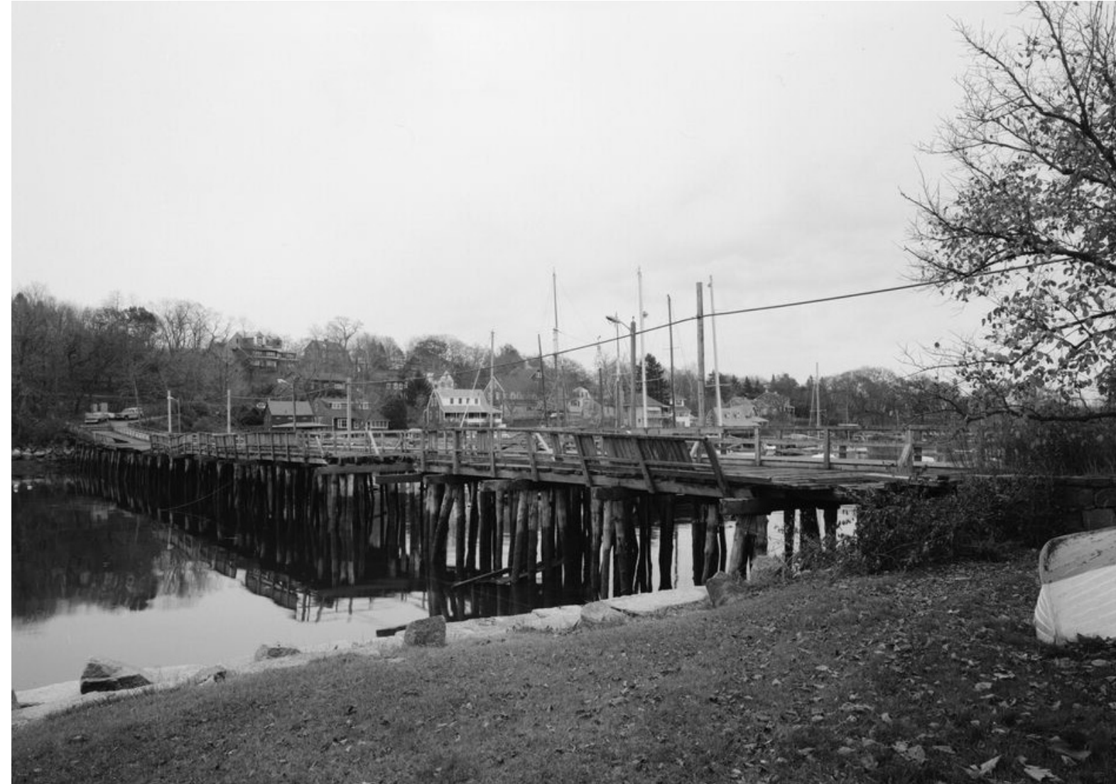
Historic American Engineering Record, Annisquam Bridge Spanning Lobster Cove Between Washington and River Streets , 1968, Photography, Historic American Buildings Survey, Library of Congress Archives
